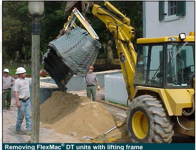
Removing FlexMac® DT units with lifting frame
