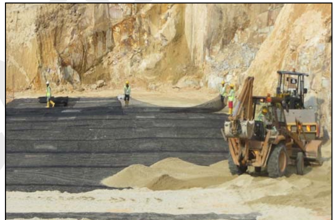
Placing MacGrid ® soil reinforcement geogrids
