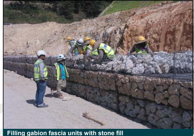
Filling gabion fascia units with stone fill
