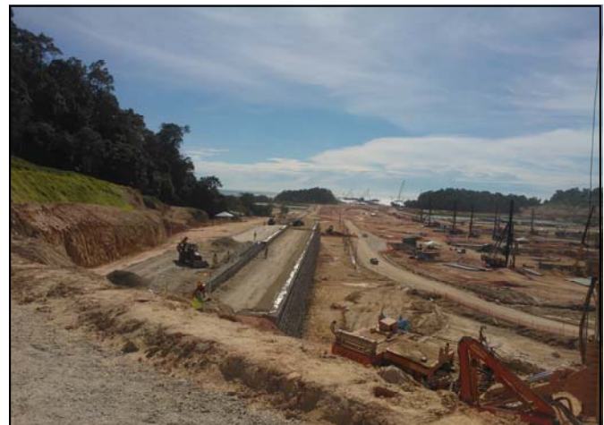
Placing and compacting backfill on the MacGrid ® geogrid
