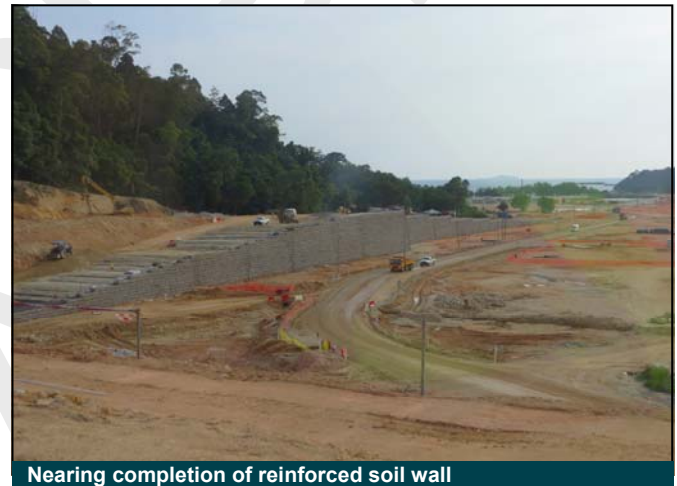
Nearing completion of reinforced soil wall
