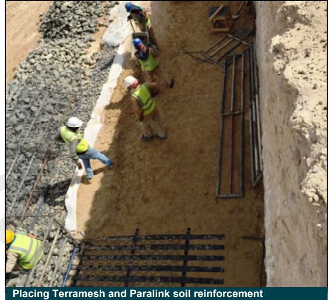
Placing Terramesh and ParaLink soil reinforcement
