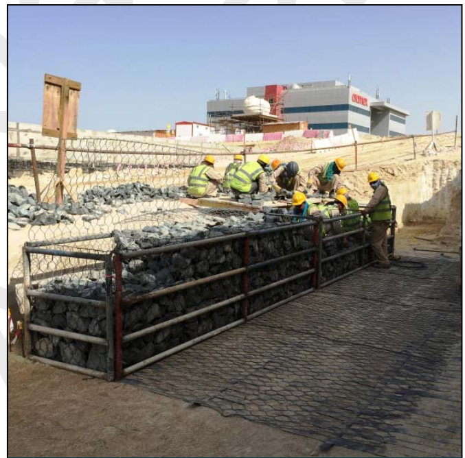
Terramesh fascia unit filling. Note Paralink geogrid in-place
