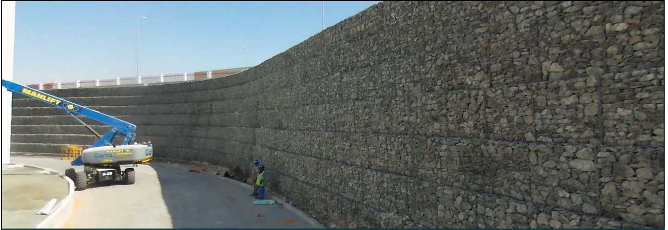
Completed structure awaiting installation of parapet crash barrier adjacent to highway
