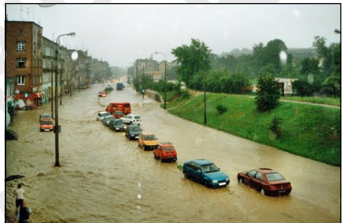
During flood - view of street showing bund before breach
