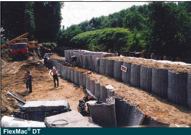
Filling the FlexMac® DT layers
