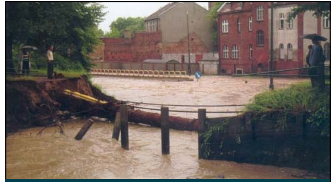
During flood. Breached embankments exposing services
