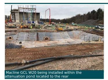
Macline GCL W20 is anchored at the crest of slopes in a trench.
