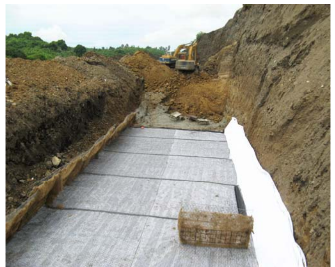
During construction Date: June 2007
