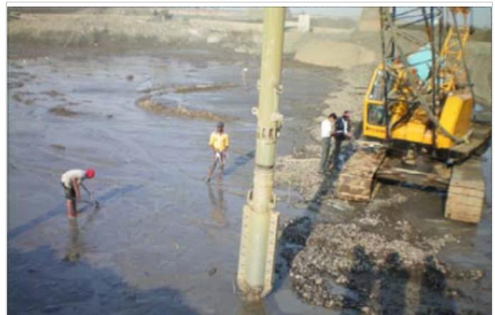
Photo-1: Installation of stone column
