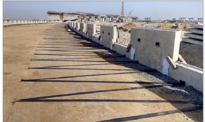
Photo 4: RS wall under construction
