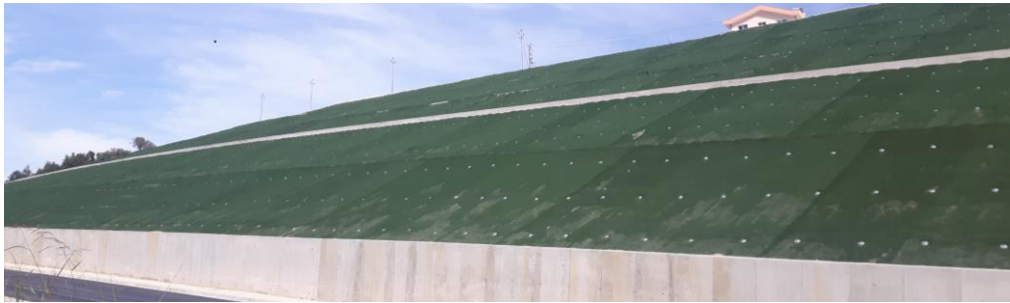
Figure 5. Soil Nailing with flexible structural facing
