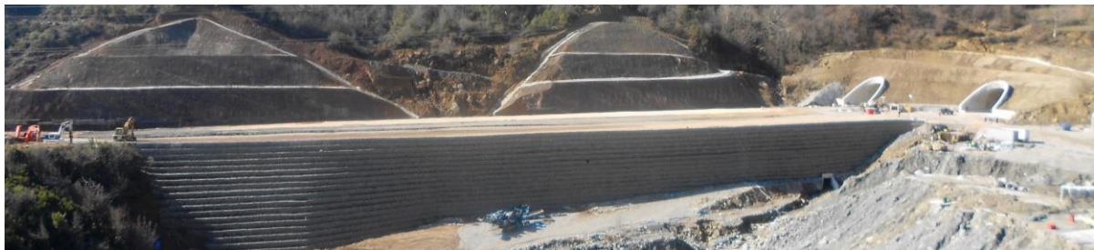
Figure 9. Terramesh System wall at the exit of Krrabe tunnel
