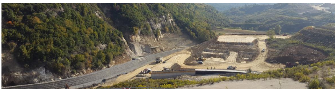
Figure 7. Terramesh System at the toe of sliding plan
