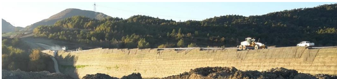
Figure 5. Green Terramesh retaining wall at section 1
