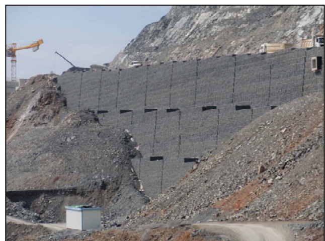
Pic. 3- the highest wall during the construction
