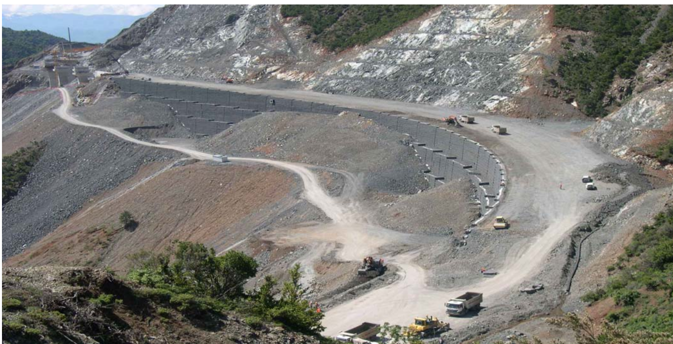
Pic.4 - overview of the highest wall
