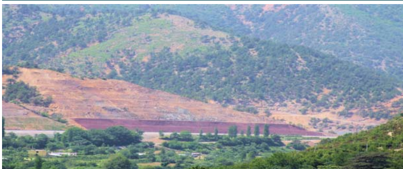
Pic. 7- Slope covered by Macmat R (brown)
