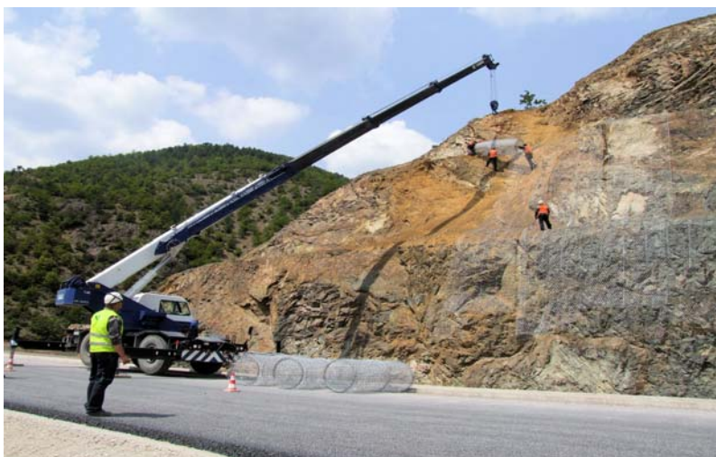
Pic.5- Steelgrid application
