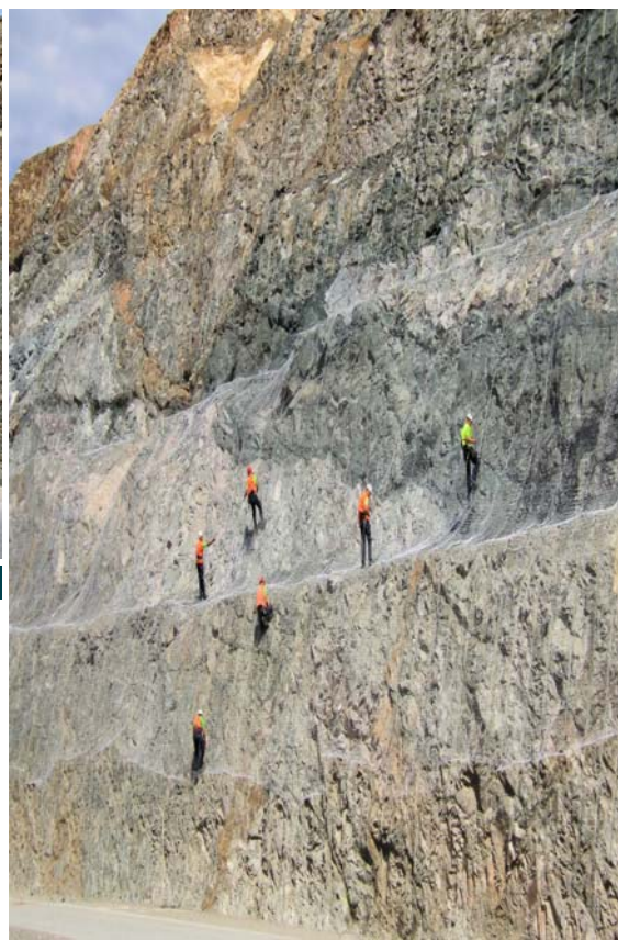
Pic. 6-Steelgrid application
