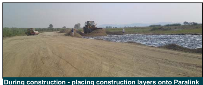
During construction - placing construction layers onto Paralink
