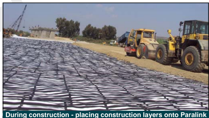
During construction - placing construction layers onto Paralink
