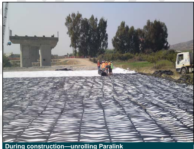
During construction—unrolling Paralink
