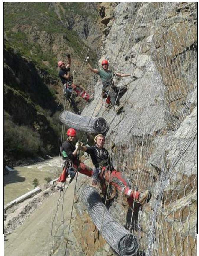
STEELGRID HR® 100 after installation
