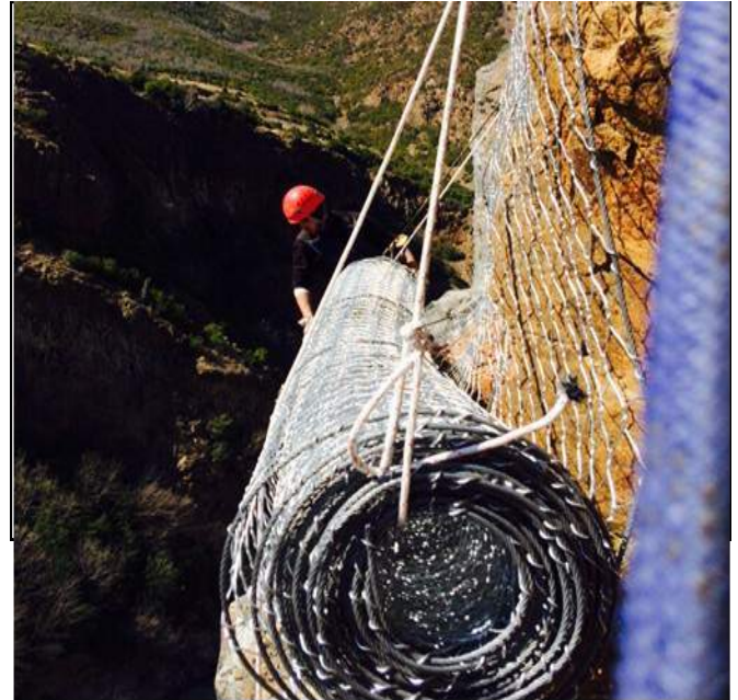
STEELGRID HR® 100 after installation
