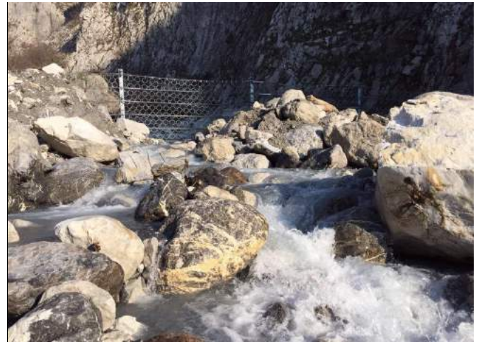
Debris Flow Barrier 200 DF after installation
