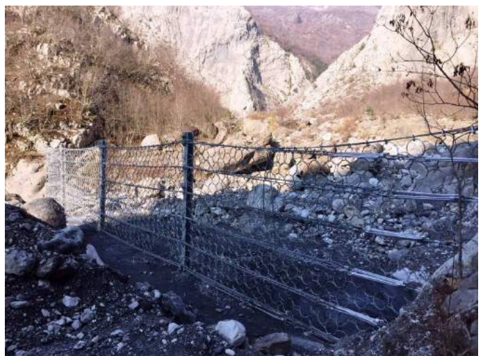
Debris Flow Barrier 200 DF after installation
