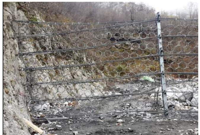
Debris Flow Barrier 200 DF after installation
