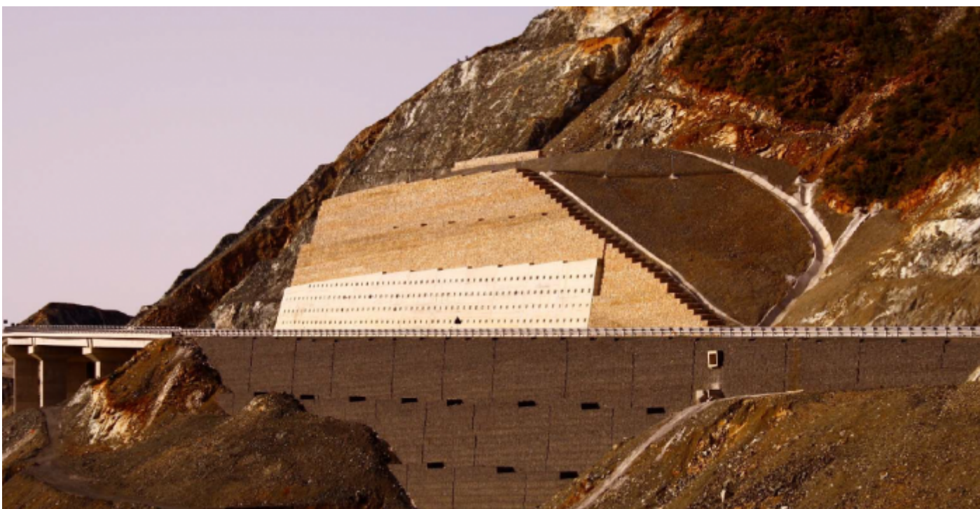
Completed reinforced soil structure with slope stabilisation measures above high
