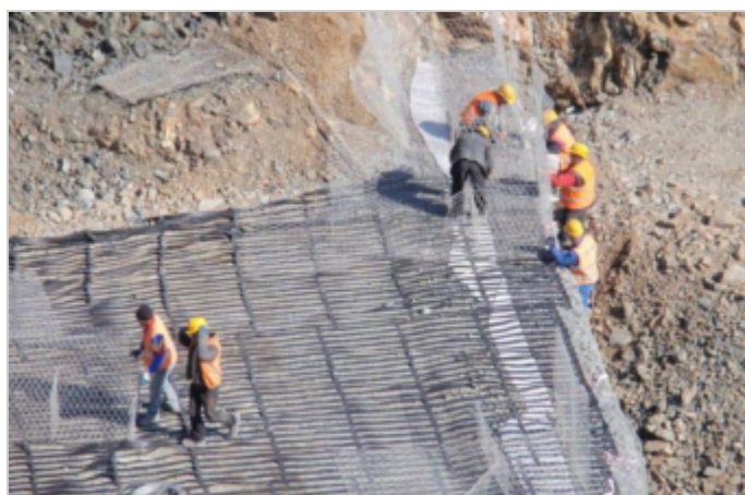
Laying Paralink primary reinforcement
