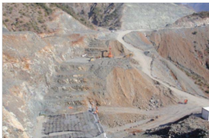
The first courses of the tallest wall being constructed
