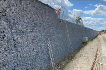
G01 wall - side view of Mineral Terramesh wall
