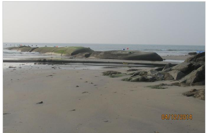
Photo 6: Silt trapped by MacTube
