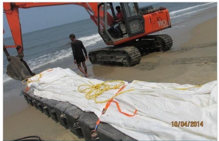
Photo 4: Transfer of tubes into the sea using pontoons
