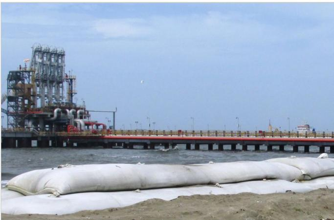
Photo 5: After construction of 500 m long protection bund structure
