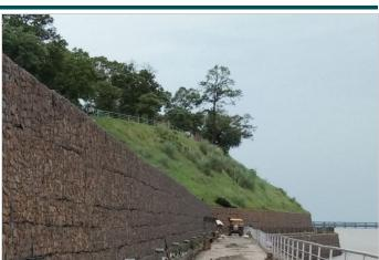
Figure 4-Vegetated surcharge slope covered with MacMat R (Paramesh wall)
