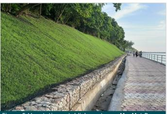
Figure 5-Vegetation establishment over MacMat R installed slope
