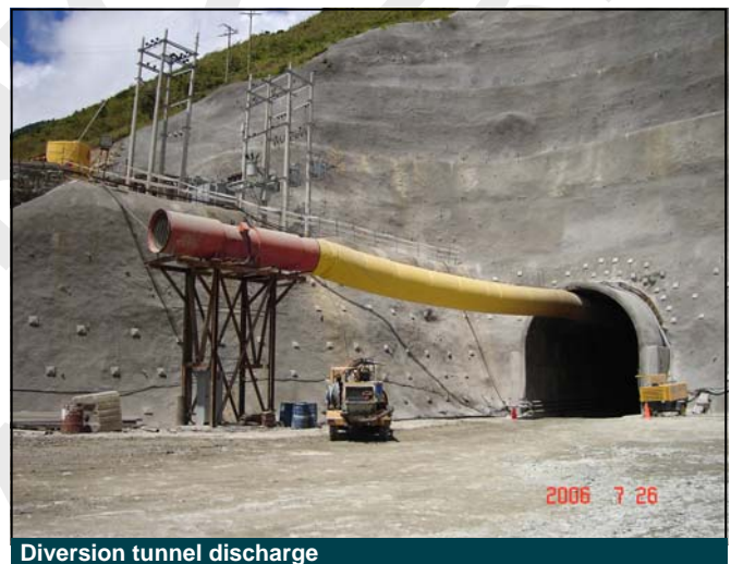
Diversion tunnel discharge
