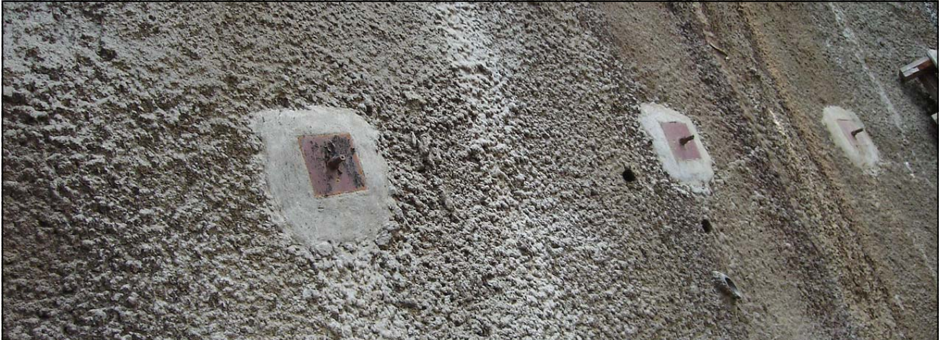
Detail of shotcrete face in conjunction with soil nails
