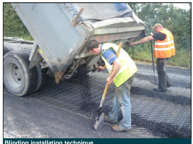
Blinding installation technique
