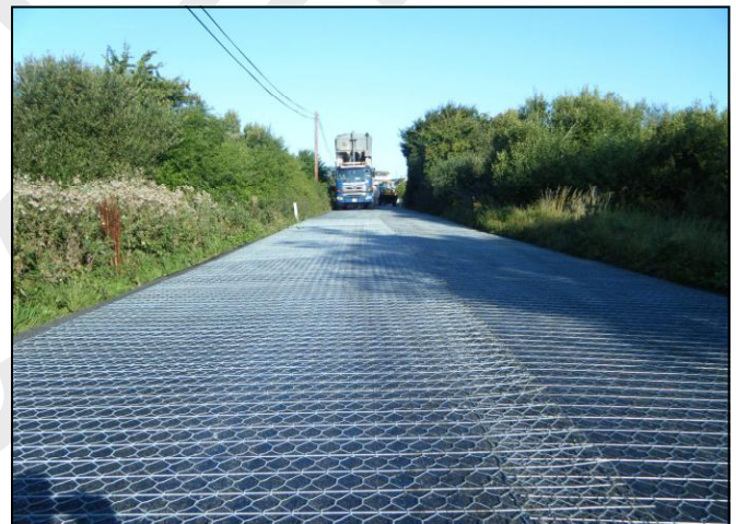
Installation of Road Mesh
