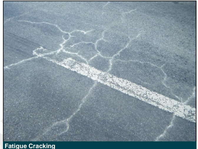
Fatigue Cracking
