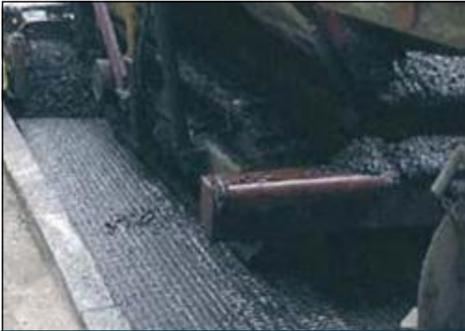
Asphalt placement onto MacGrid
