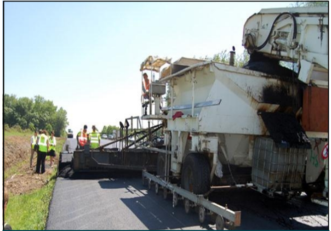
Asphalt placement onto MacGrid
