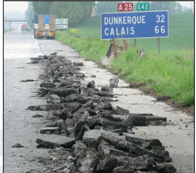
Removal of fatigued surface layer
