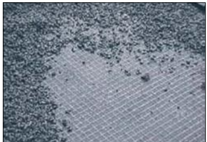
MacGrid ARG placed on prepared surface
