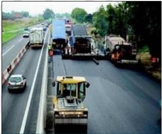
The works progressing
