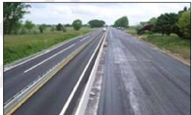
Surface ready to receive bond-coat and MacGrid
