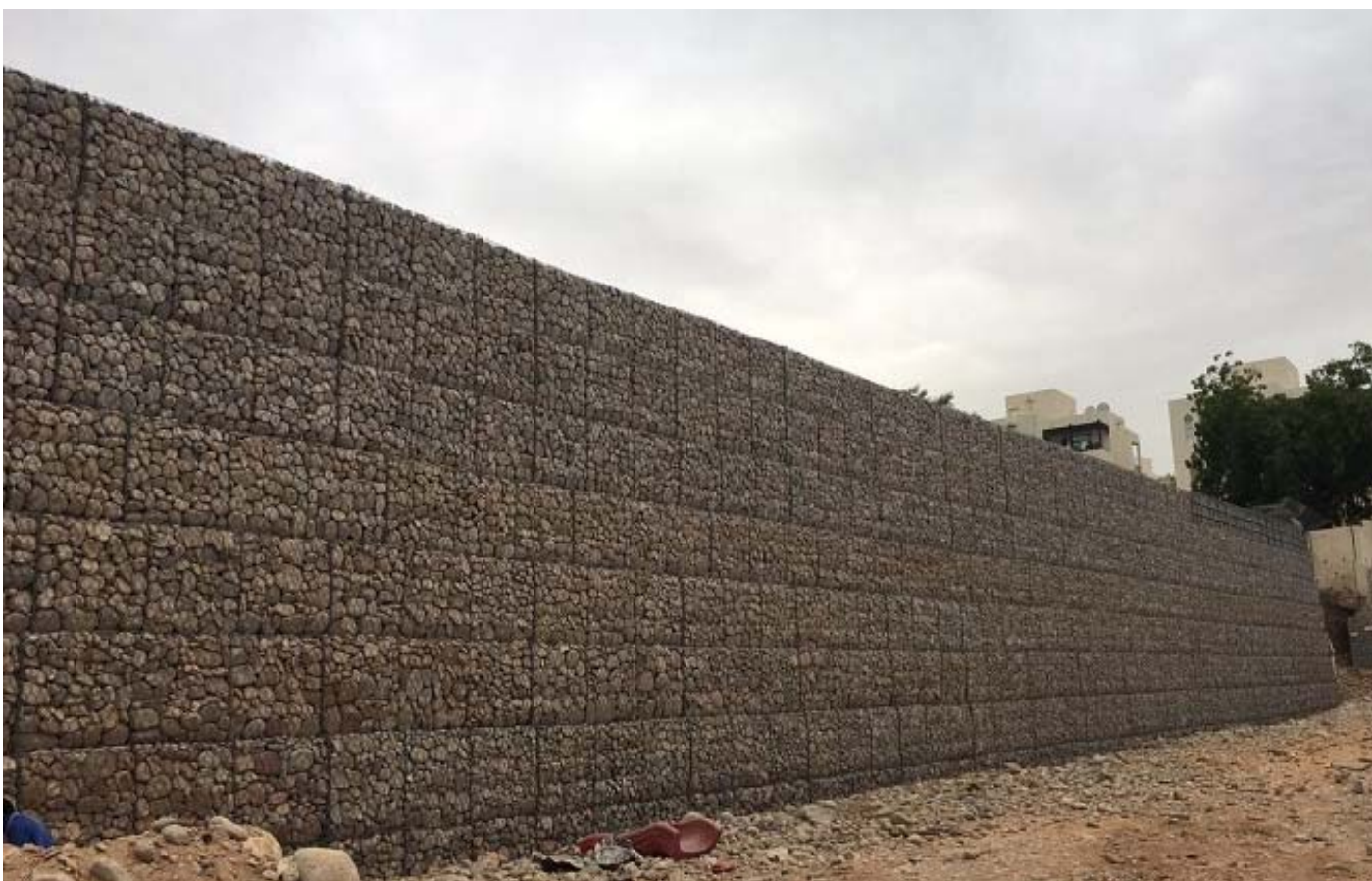
ParaMesh Wall (NorthSide) - After Construction
