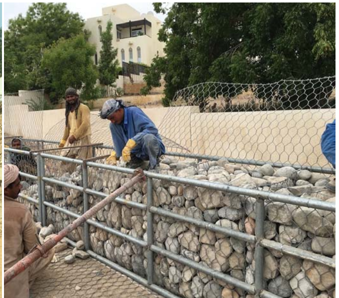
ParaMesh Wall Under Construction
