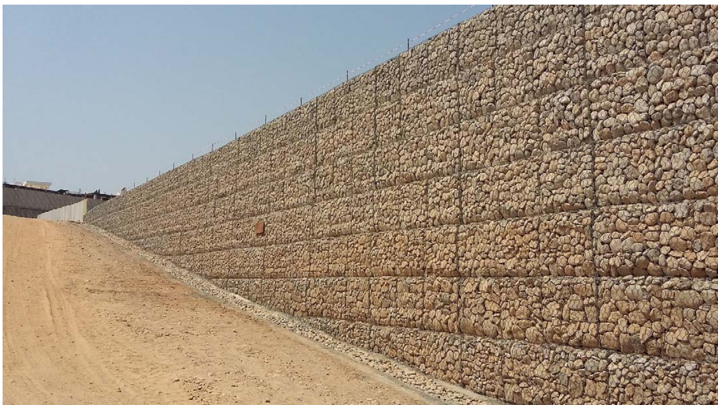
ParaMesh Wall (East Side) - After Construction
