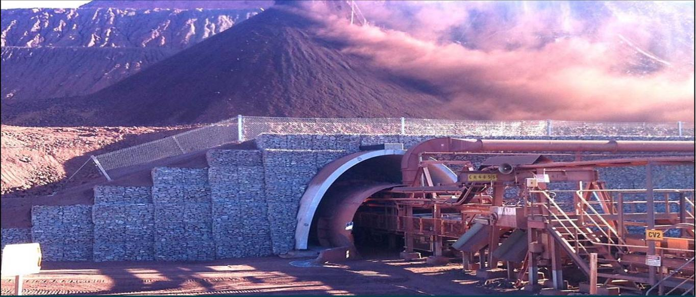
The completed 7m high mass gravity gabion north wall
