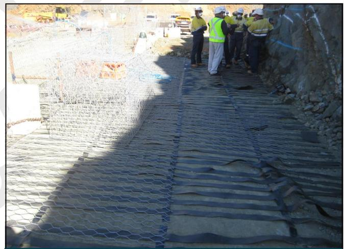
During construction - laying Paralink & Terramesh
