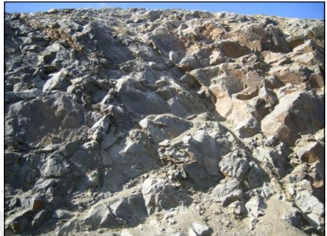
Unstable blasted slope requiring protection
