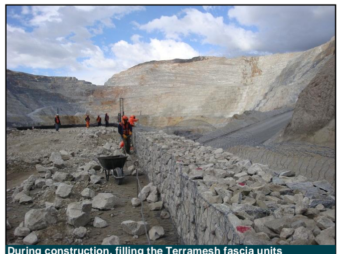
During construction, filling the Terramesh fascia units
