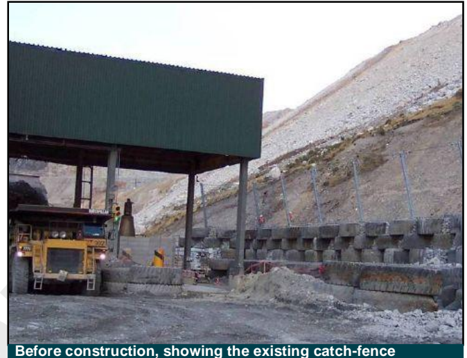
Before construction, showing the existing catch-fence
