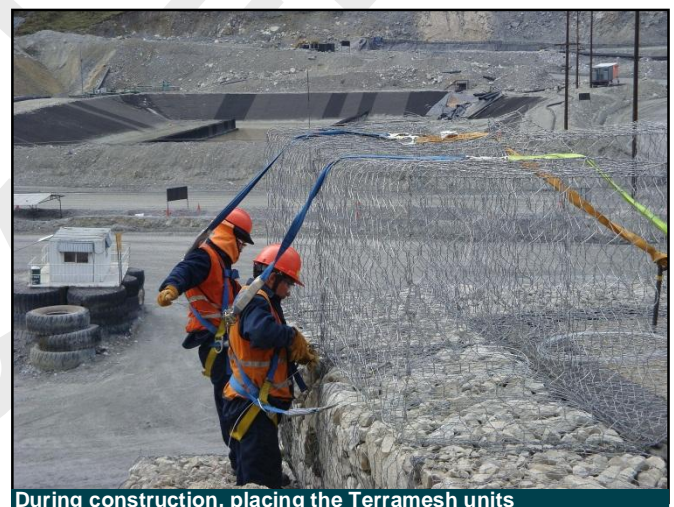
During construction, placing the Terramesh units
