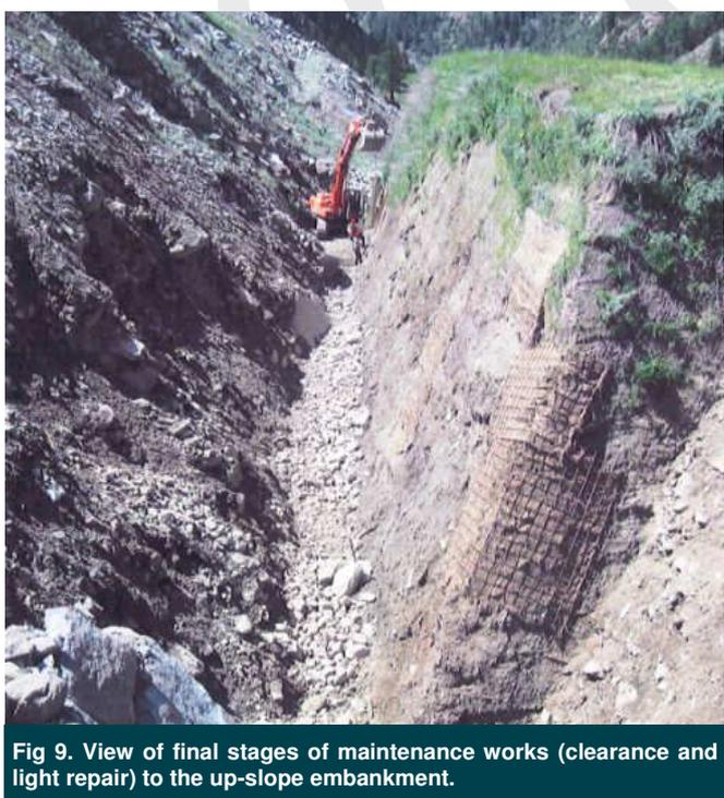
Fig 9. View of final stages of maintenance works (clearance and light repair) to the up-slope embankment.
