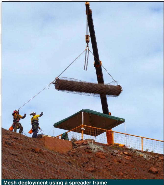
Mesh deployment using a spreader frame
