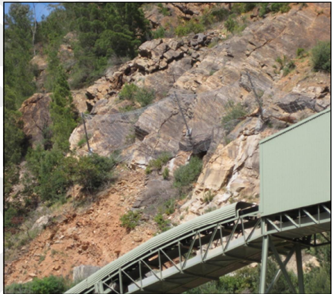
Completed barrier installation works Date: Oct 2008
