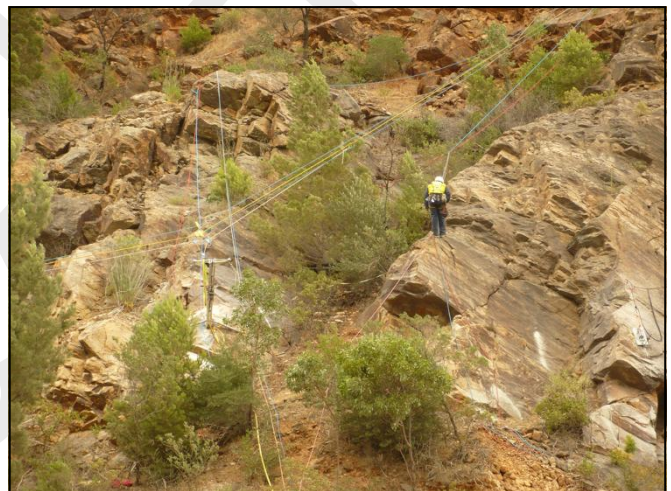
Drilling for the anchors
