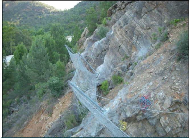
Completed barrier installation works Date: Oct 2008
