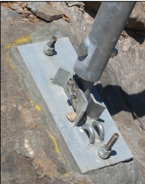
Barrier foot-plate detail Date: Oct 2008
