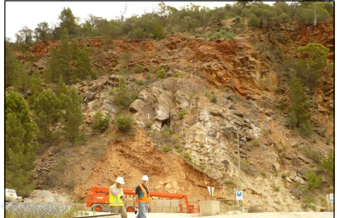
Drilling for the posts
