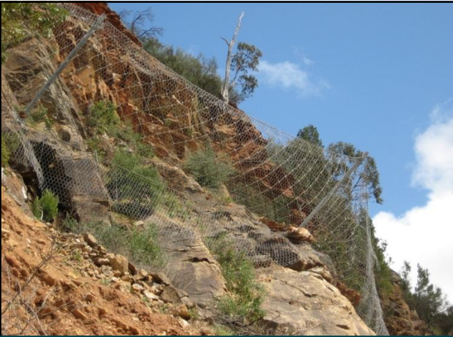
Completed barrier installation works Date: Oct 2008
