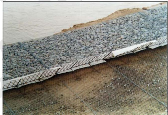
During installation—note geotextile at face of unit
