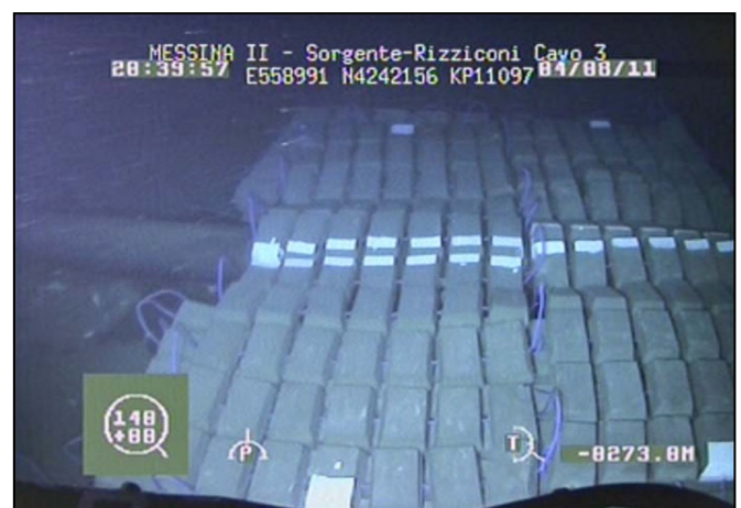
Installed ACBM Mattresses
