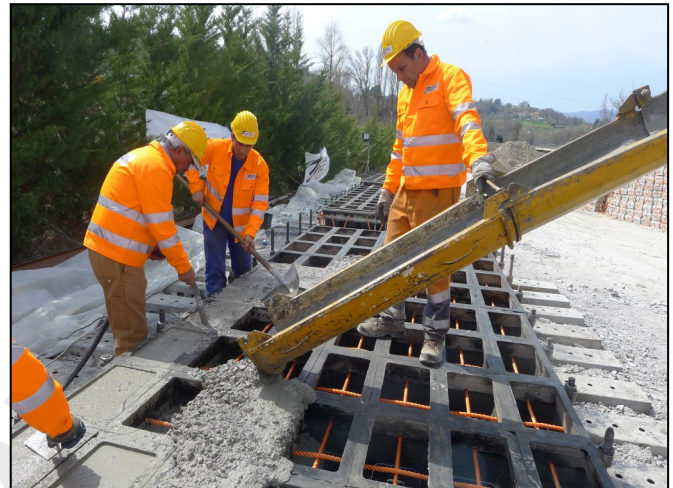
ACBM mattresses casting operations
