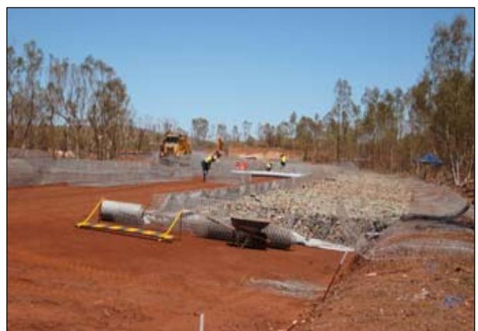
Assembly and filling of the Gabions
