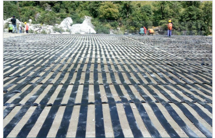
Photo 4: Laying of ParaLink
