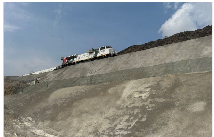
Completed: Shotcrete covered slope reinforced with Paragrid geogrid
