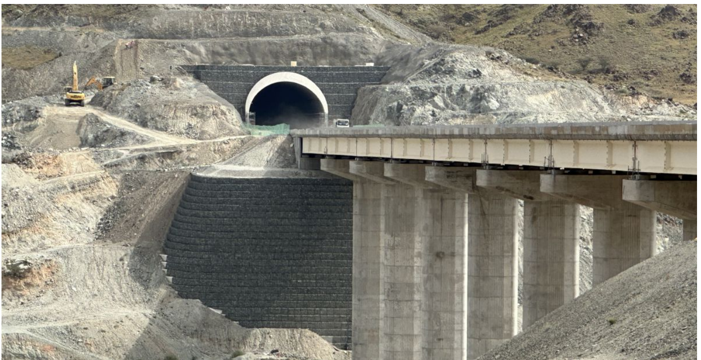
Completed: Terramesh MSE wall at bridge and tunnel portal locations.
