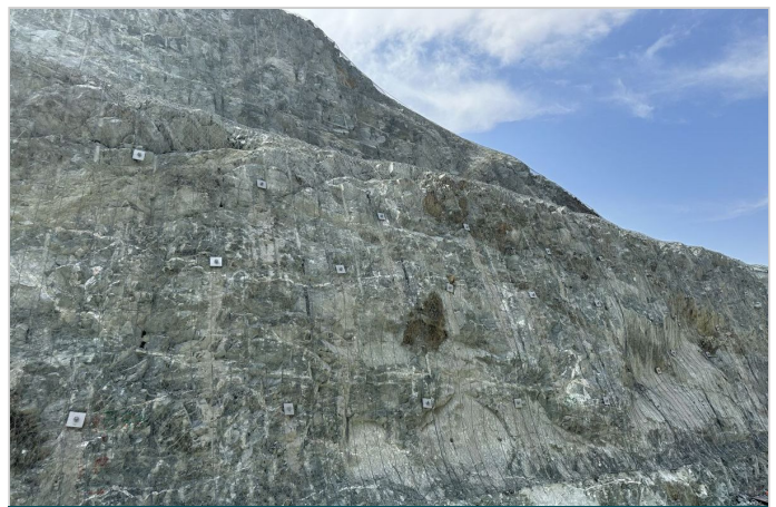
Completed: Secured drapery with Steelgrid HR mesh
