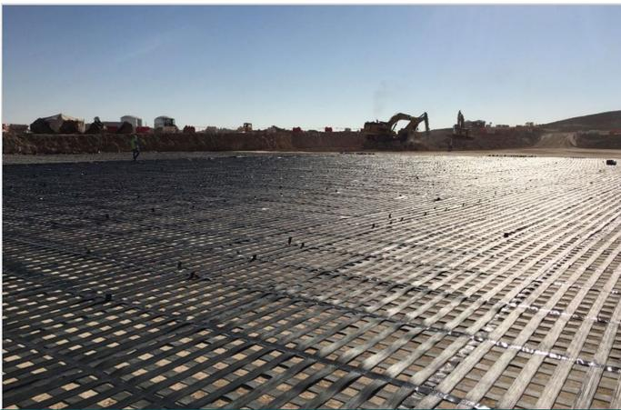
During construction: high strength Paralink geogrid laying in progress
