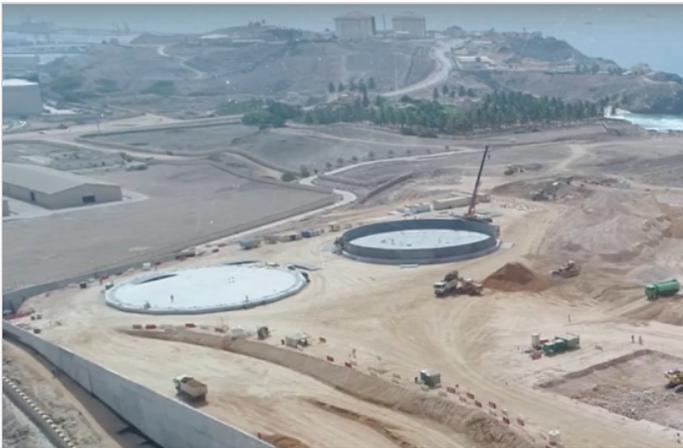
During construction: concrete tank foundation in progress
