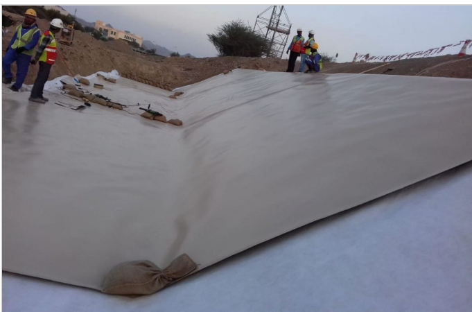
During construction: Beige colour HDPE geomembrane lining layer installation
