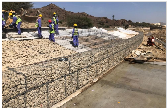
During construction: Polimac coated gabion mattress installation on side slopes
