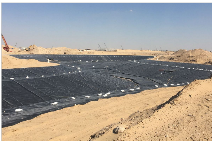
During construction: HDPE geomembrane water proofing layer installation
