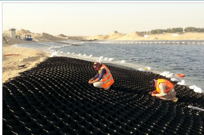
During construction: Macweb geocell installation on side slopes
