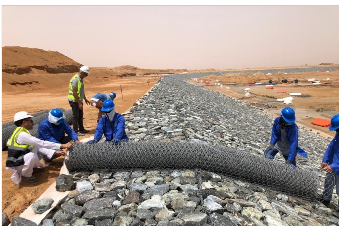
During construction : unrolling of closing lid in progress
