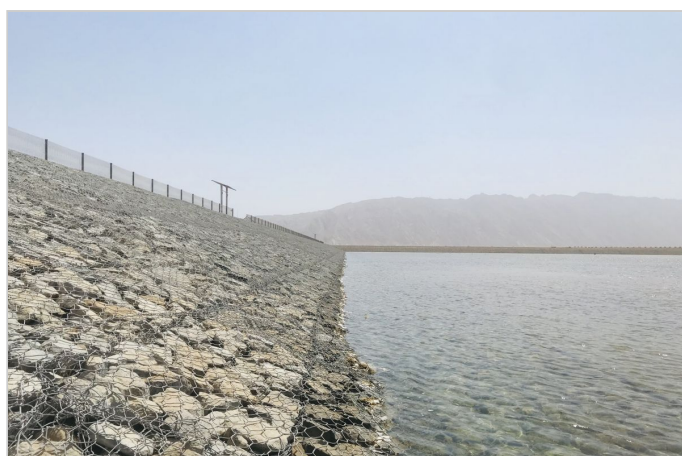
Completed pond : water level rising after stopping de-watering
