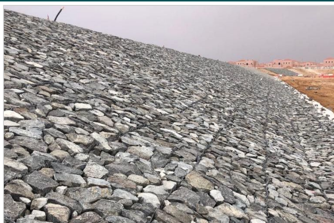
During construction : filled gabion mattress before placement of closing lid
