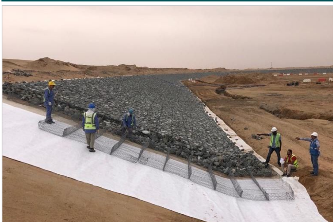
During construction : gabion mattress filling in progress
