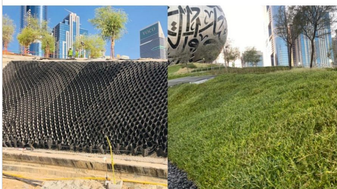
During construction: Macweb geocell (before & after vegetation growth)
