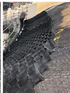
Macweb Geocell & Steel Cable installation
