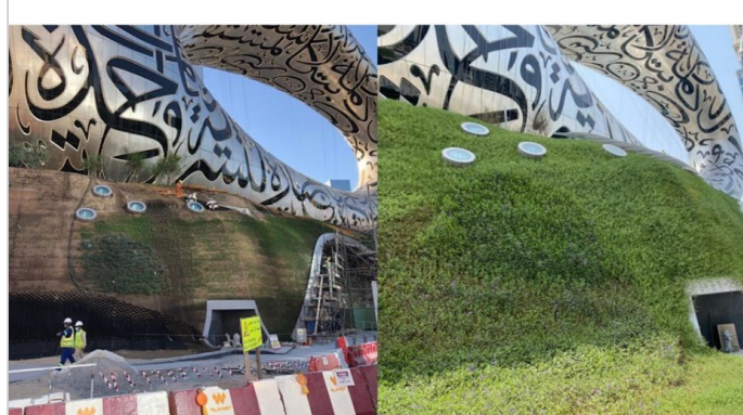
During construction: Green Terramesh soil slope (before & after vegetation)
