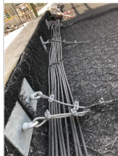
Macmat HS & Concrete Anchor Installation
