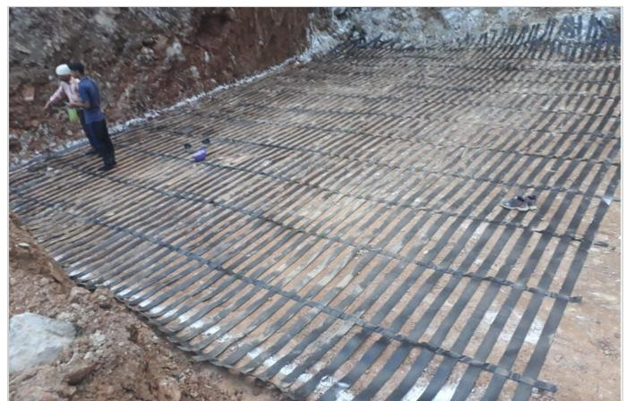
Photo 2: During construction- Laying of ParaLink
