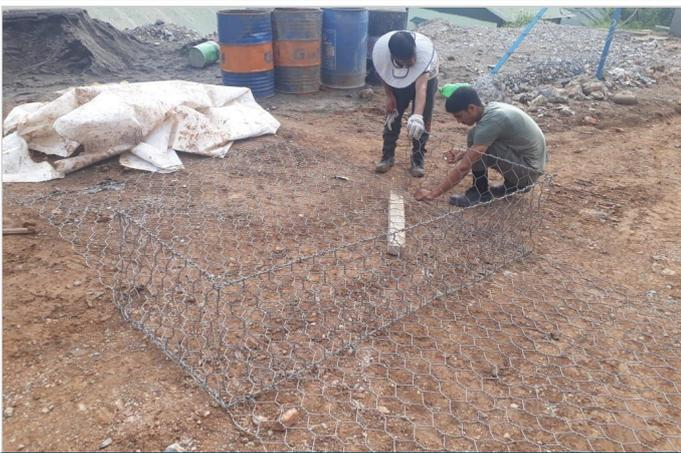
Photo 3: During construction- assembly of Terramesh units
