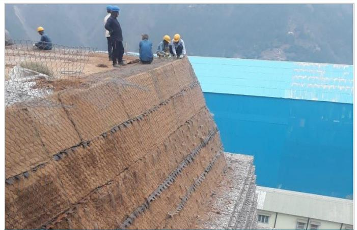
Photo 5: Installation of Green Terramesh units
