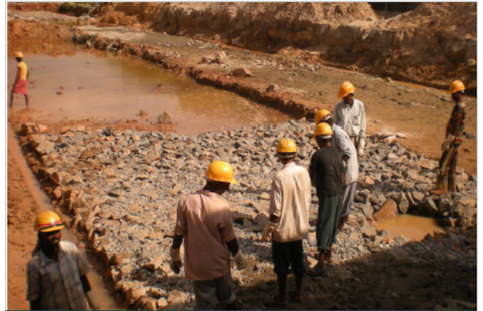
Photo 4: Placement of boulders
