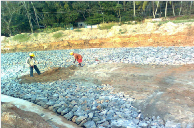
Photo 3: Laying of boulders at foundation levels on top
