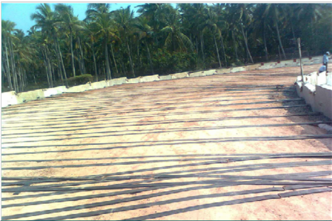
Photo 5: Installed Paraweb
