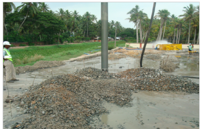
Photo 2: Installation of stone column
