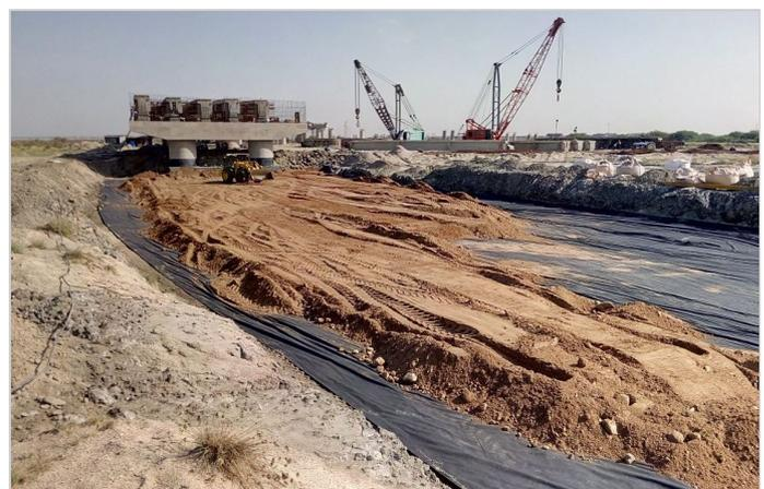
Photo 2: Placement of sand and geotextile
