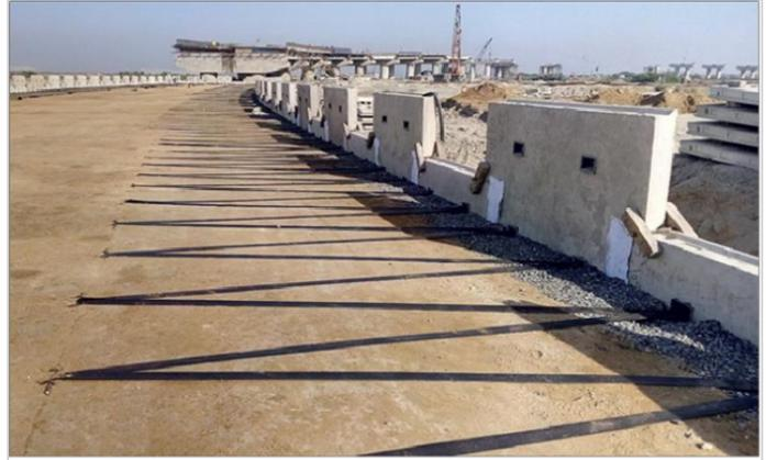
Photo 4: RS wall under construction
