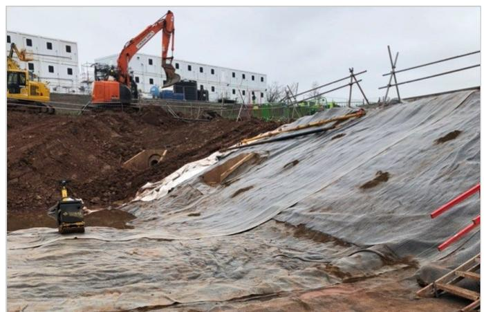
Macline GCL W20 installed and covered with minimum 300mm covering topsoil.
