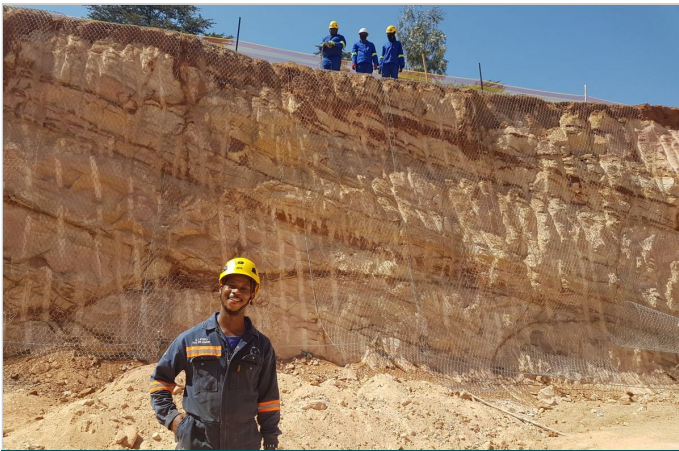
Installation of the DT Mesh to the Eastern Slope
