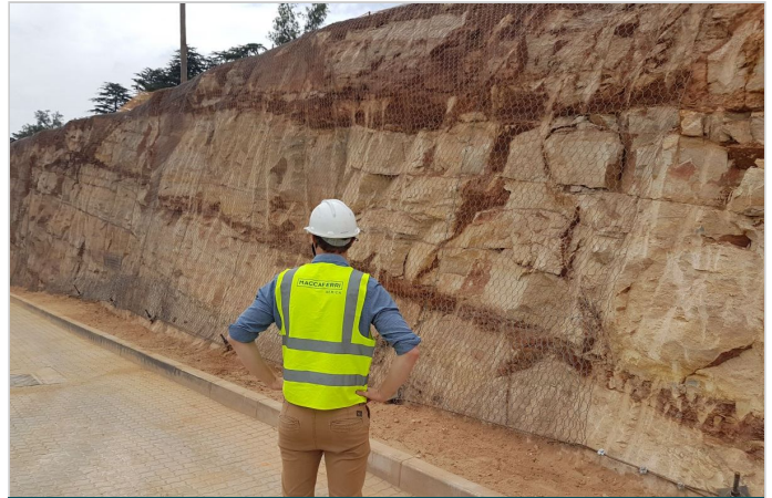
Installation of the DT Mesh to the Eastern Slope
