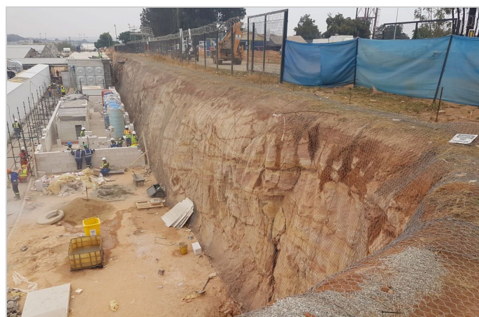
Installation of the DT Mesh to the Northern Slope
