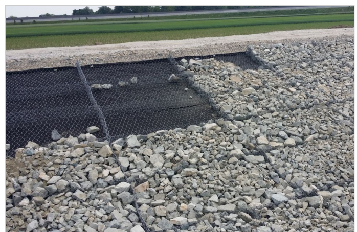
During the installation: stone-filling operation
