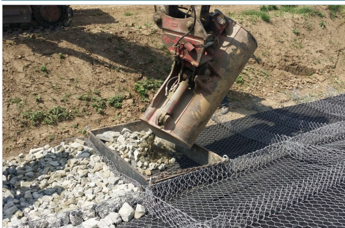
Installation phase: stone-filling operation
