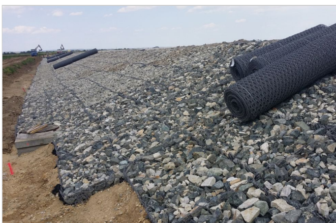
During the installation: closing of the units with DT-net
