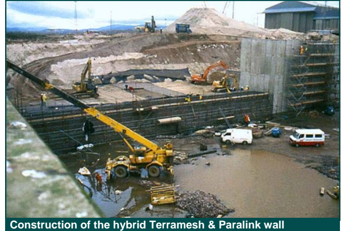
Construction of the hybrid Terramesh & Paralink wall
