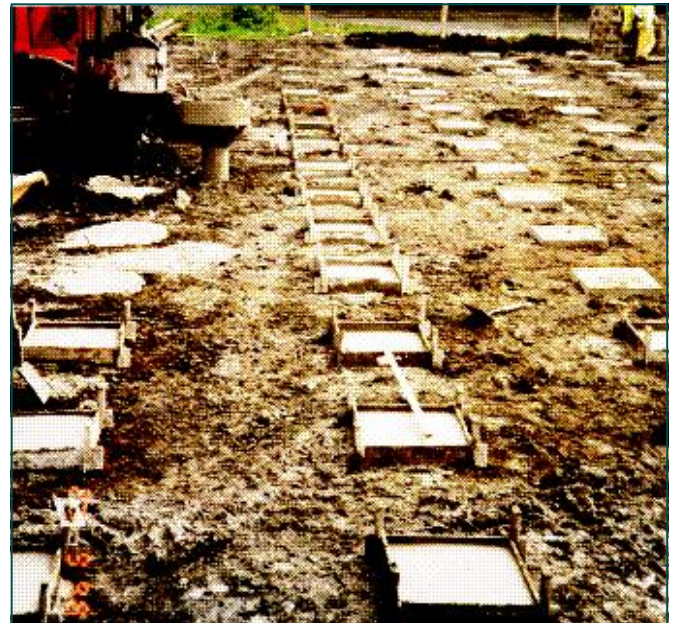
Preparation of pile caps
