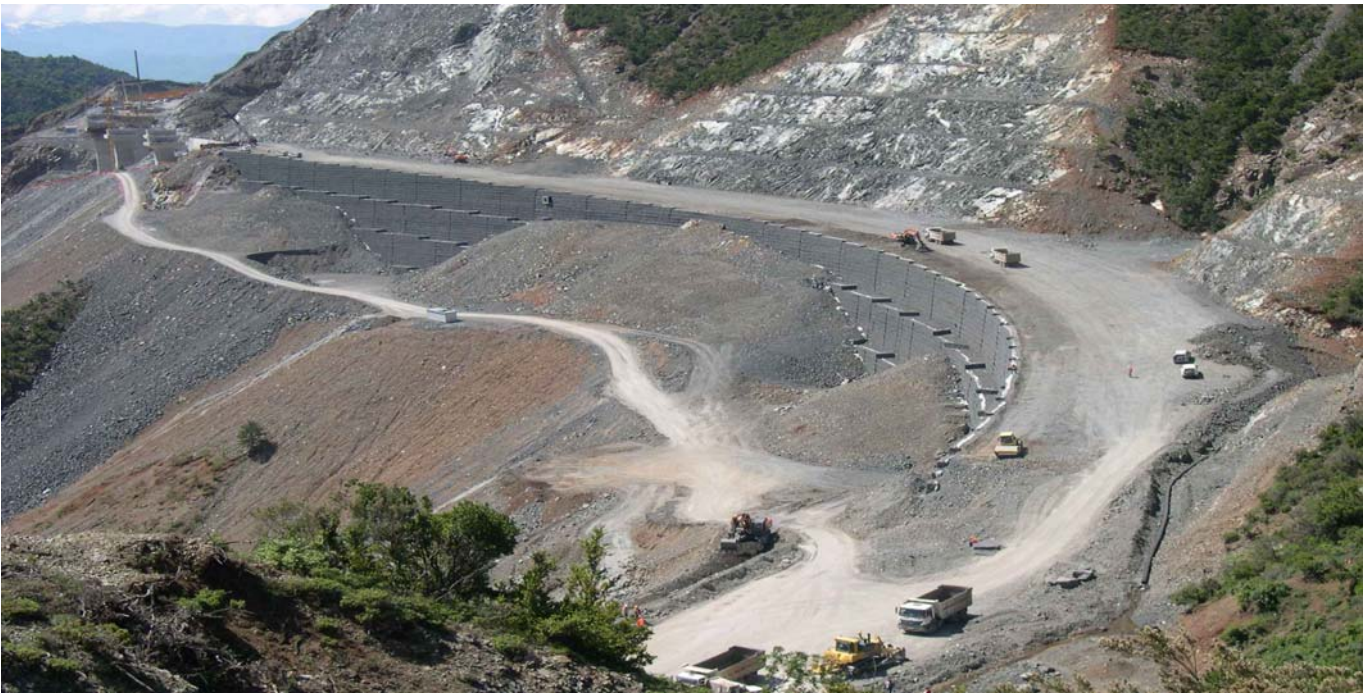
Pic.4 - overview of the highest wall
