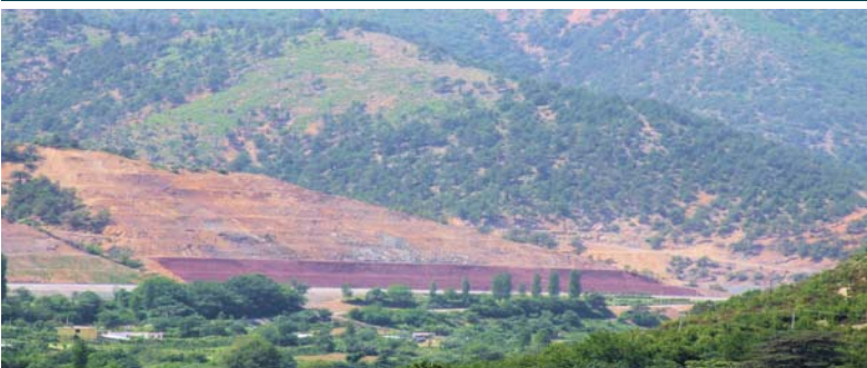
Pic. 7- Slope covered by Macmat R (brown)
