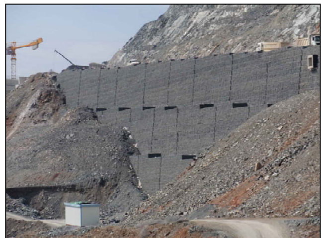
Pic. 3.- the highest wall during the construction
