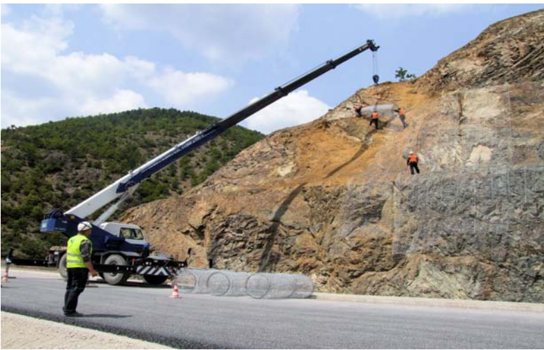
Pic.5- Steelgrid application
